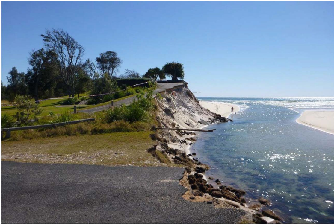
Figure 5-3 Entrance channel migration northwards and erosion of the dunal profile prior to construction of the existing coastal protection works
