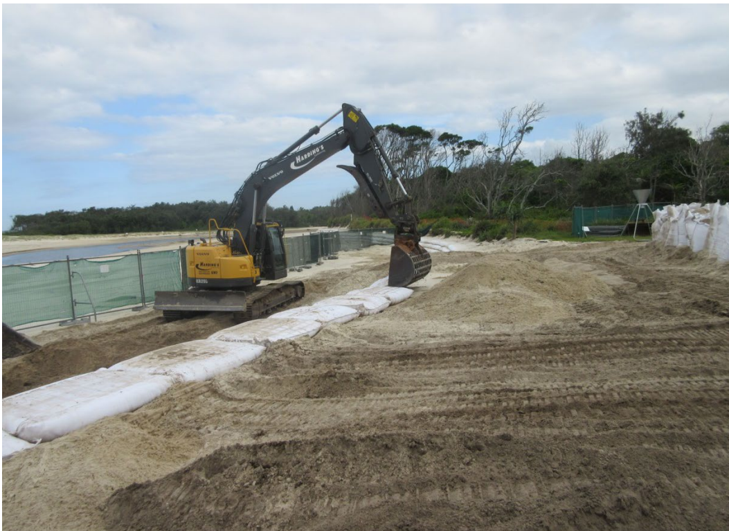
Figure 2-4 View showing excavator positioning geobags in the structure (March 2015)
