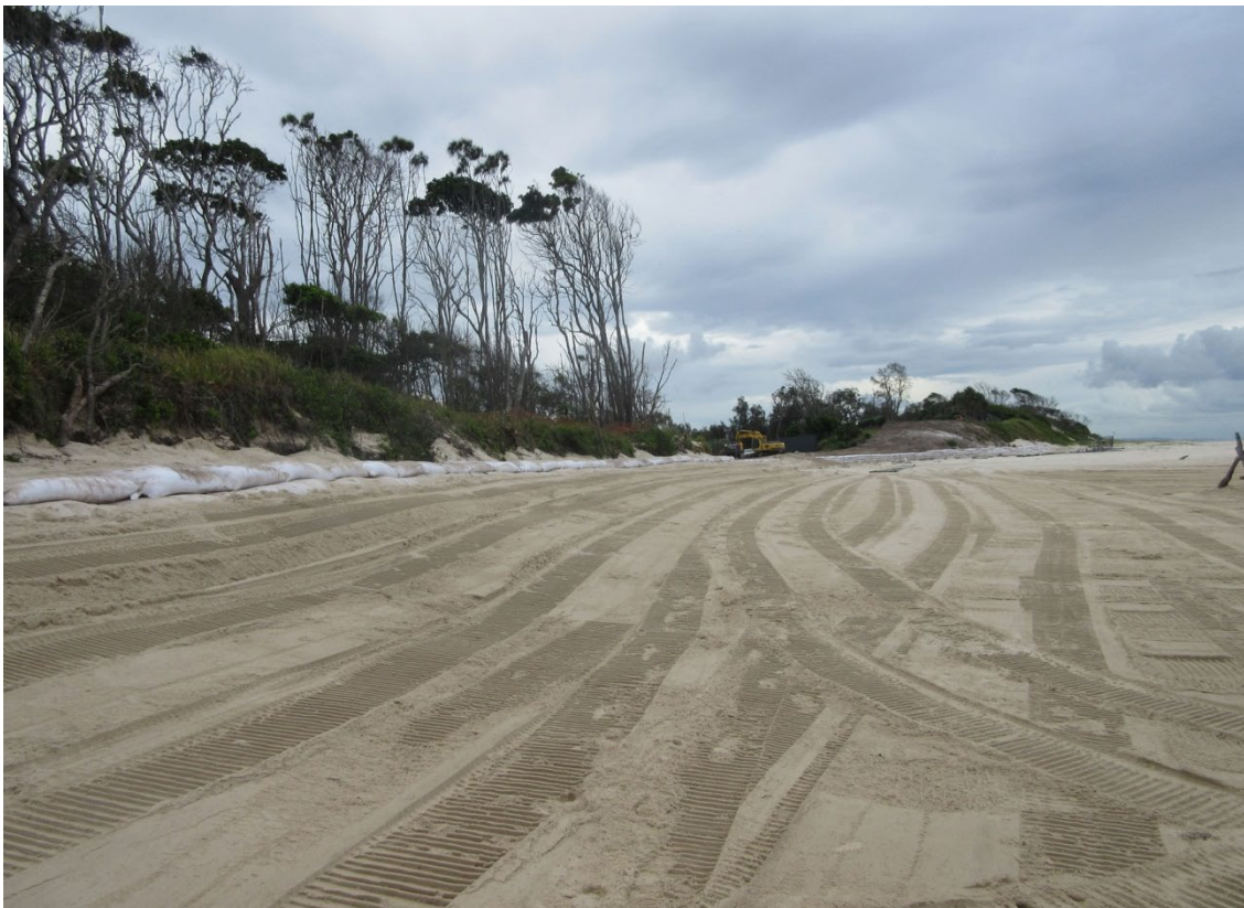
Figure 2-6 Reshaping and grooming of the beach in front of the protection works at completion (March 2015)
