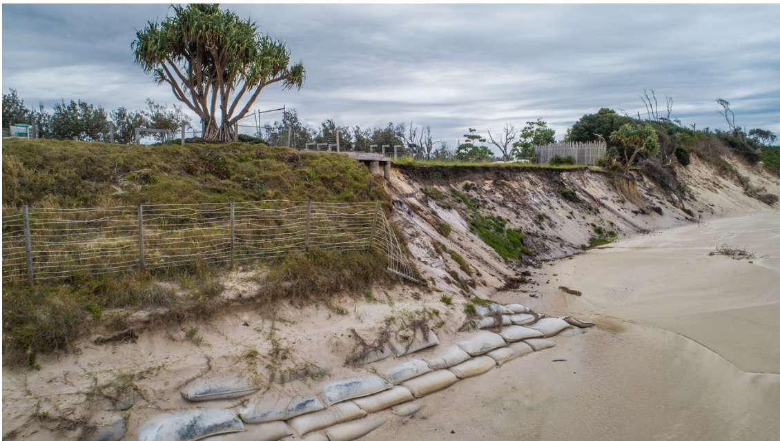
Figure 3-1 Erosion immediately north of the existing geobag structure showing steep dune escarpment and undermining of foreshore assets (20 October 2022)
