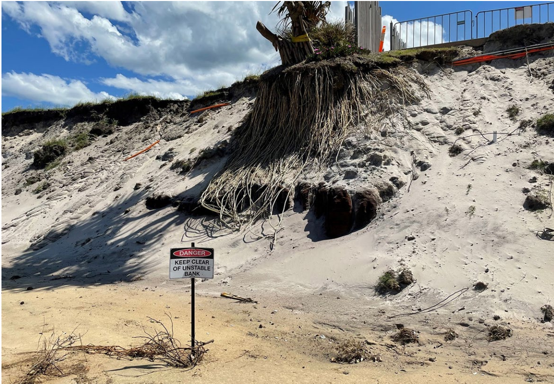
Figure 3-4 Warning signage 'Danger – Keep Clear of Unstable Bank' near the base of the erosion escarpment north of the geobag structure. The escarpment is at or near the natural angle of repose and is a potential public safety risk to users of the beach (25 October 2022)
