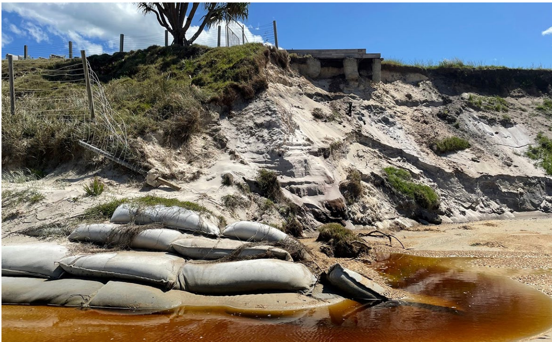
Figure 3-3 Close up view of the northern limit of the existing geobag structure and adjacent erosion (25 October 2022)
