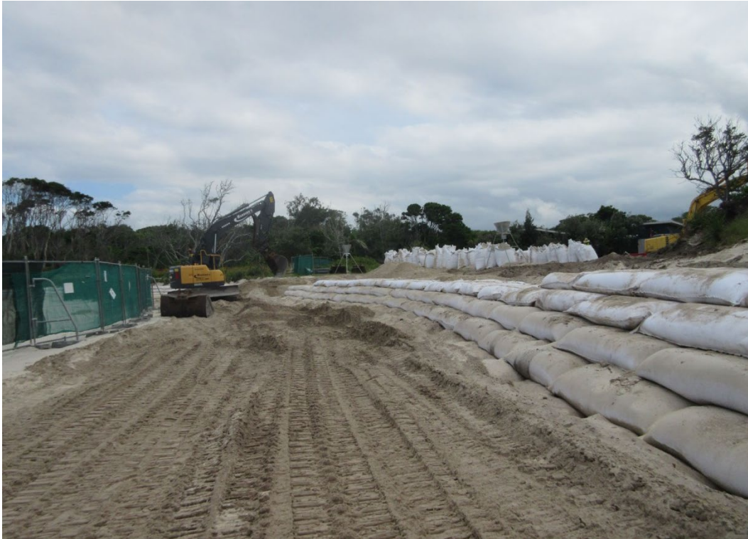
Figure 2-5 View of a section of the completed coastal protection works five units high (March 2015)
