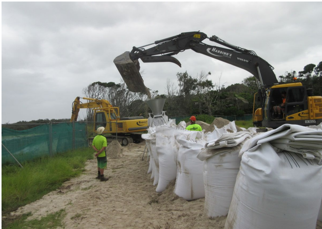
Figure 2-2 Filling geobags with sand from the imported sand stockpile using an excavator (March 2015)
