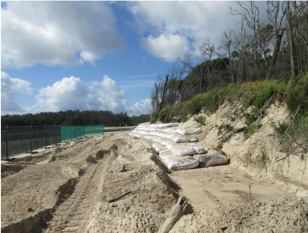
Figure 2-3 View looking southwards during construction showing the prepared foundation for the protection works and the rows of geobags (March 2015)
